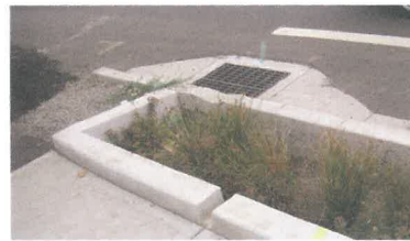
Swales, like this one in Portland, Oregon, are low-lying planting beds engineered to capture and retain storm water.
