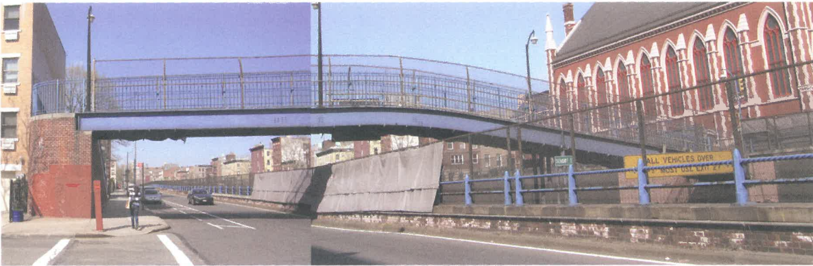
The existing Summit Street bridge rises 14' above southbound Hicks Street before reaching the BQE.
