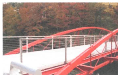
Top, a box truss bridge in Manchester, England, equipped with acoustic panels. Bottom, a pony truss bridge in Indianapolis. Connections could be completed with either kind of truss, or with a combination of multiple types. Bridges of different types, colors, or details could impart a sense of whimsical individuality to the crossings.
