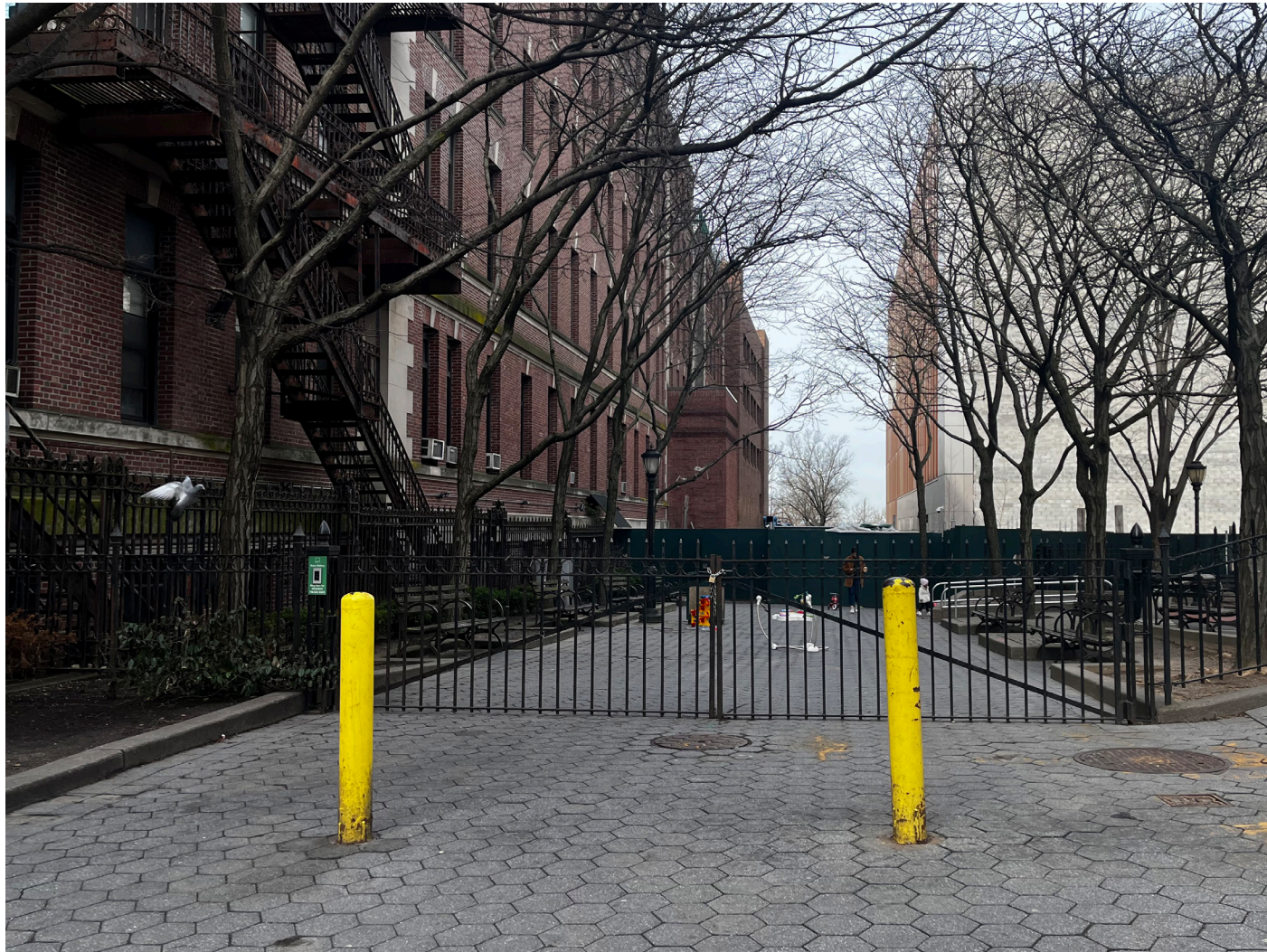
1. Pacific Street Entrance Gate & Bollards via Henry Street
